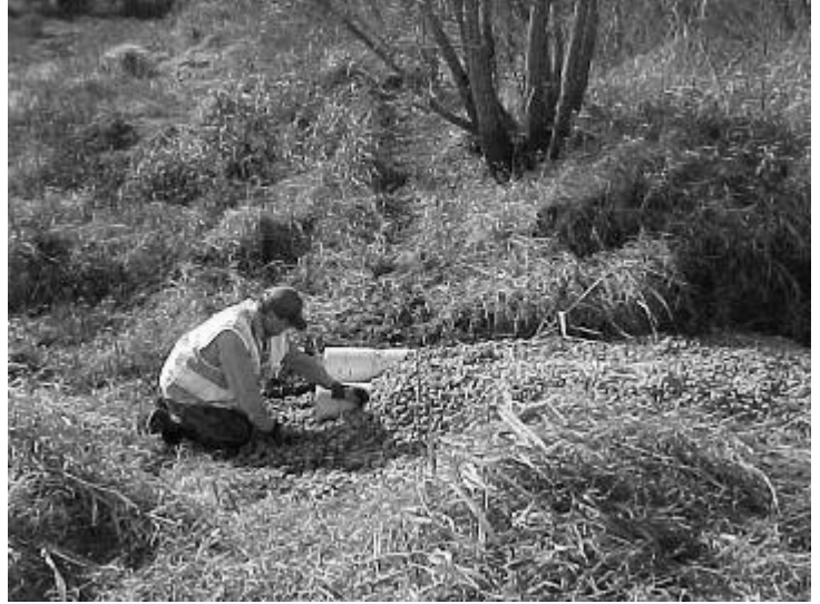
Jim Lilienthal of the DNR puts finishing touches on the man-made beaver dam on the east side of Lake Shamineau in preparation for the installation of the Clemson Levelers.
